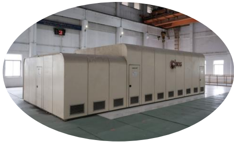
Waste heat generator
