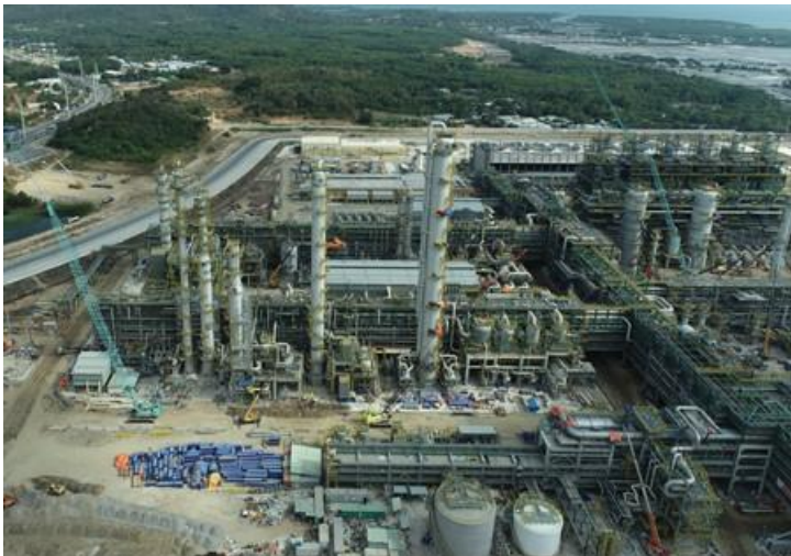
Completion of Main Columns
