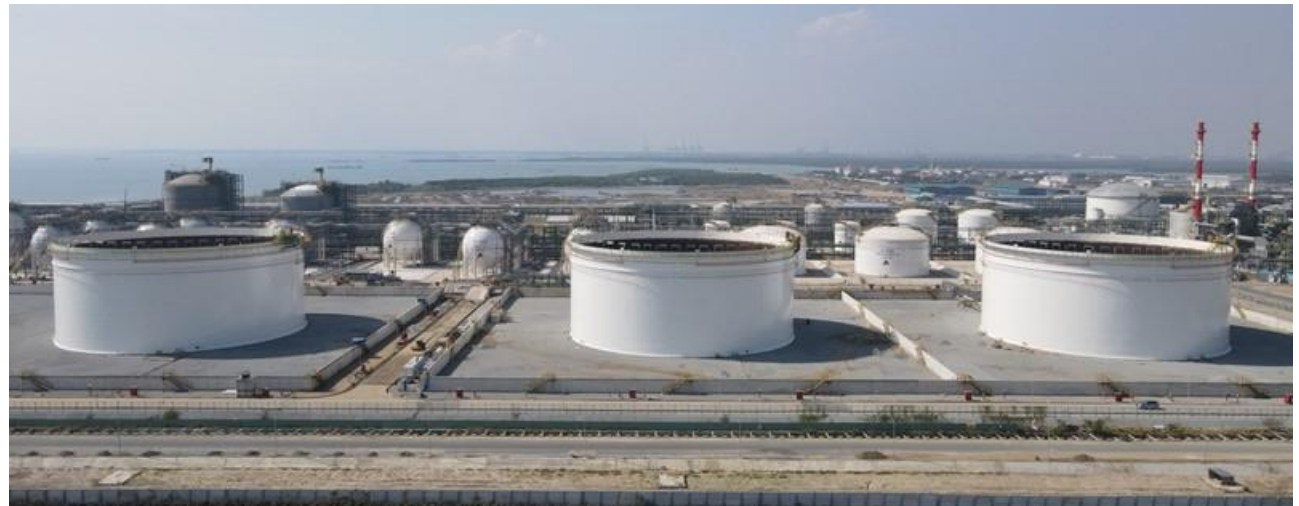
Naphtha Storage Tanks (Part of Flexible Feedstock)
