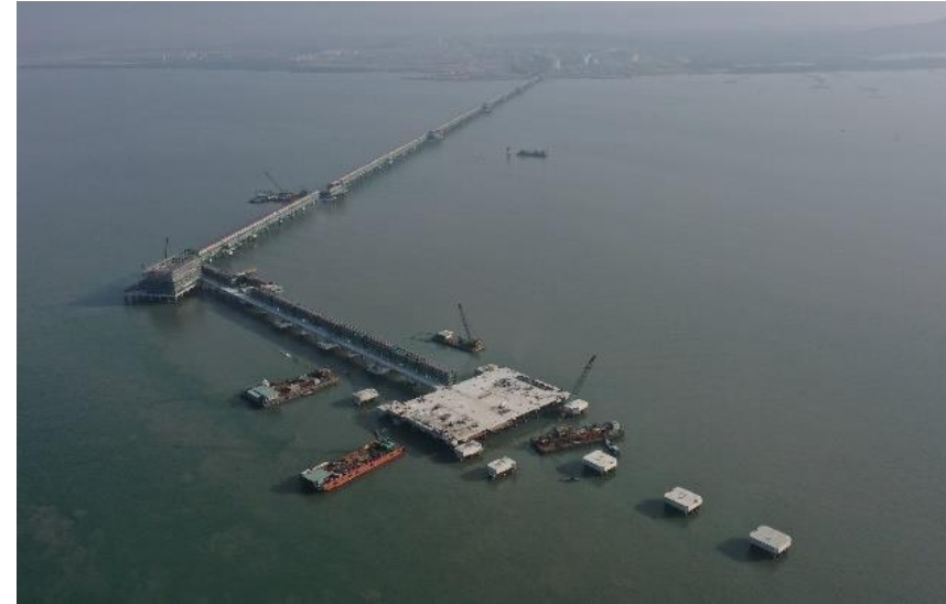
Trestle Modular Piperack at Hydrocarbon Jetty
