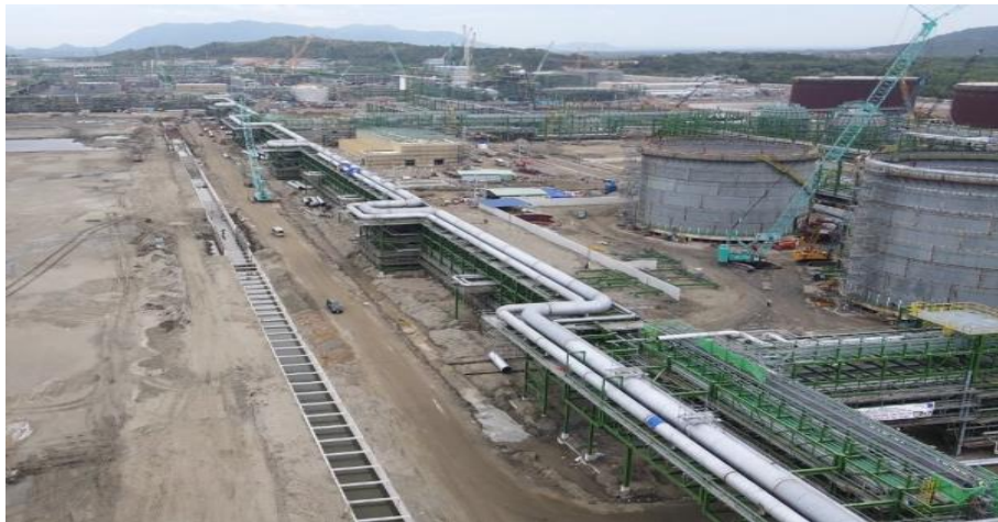
Interconnecting Piperack
