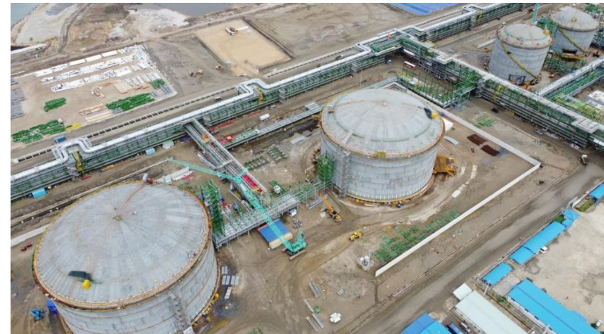
Roof Air Raising of Tanks
