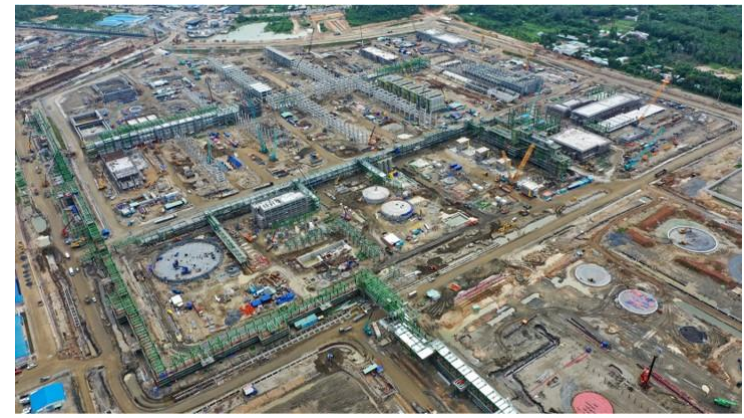
Foundation and Underground Piping works at Olefins and Central Utilities area
