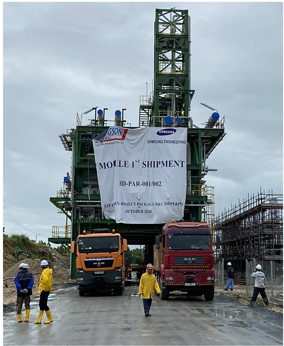
1st Module Unloading at Construction Jetty
