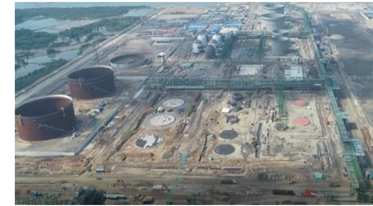
Tanks and Pipe Rack erection at Tank Farm Area
