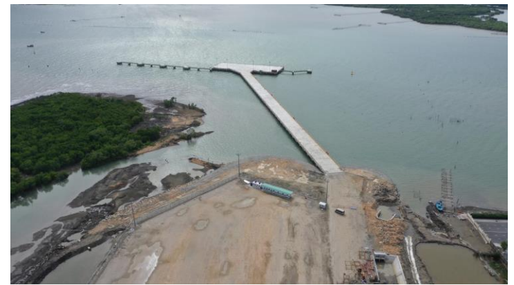
Construction Jetty Ready for Operation
