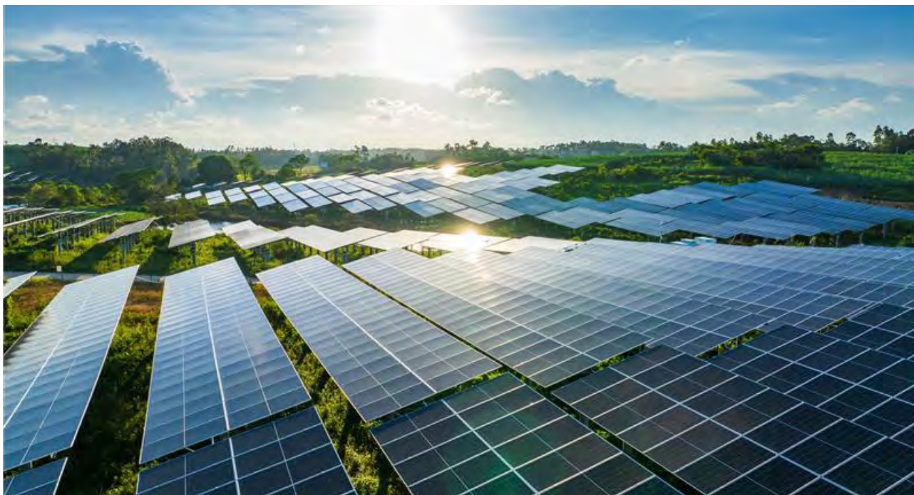
ONNEX Solar Farm
