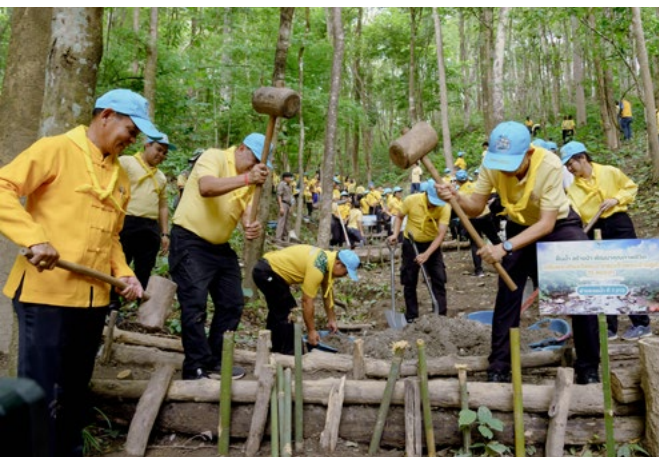
SCG unites volunteers to build check dams for water conservation.
