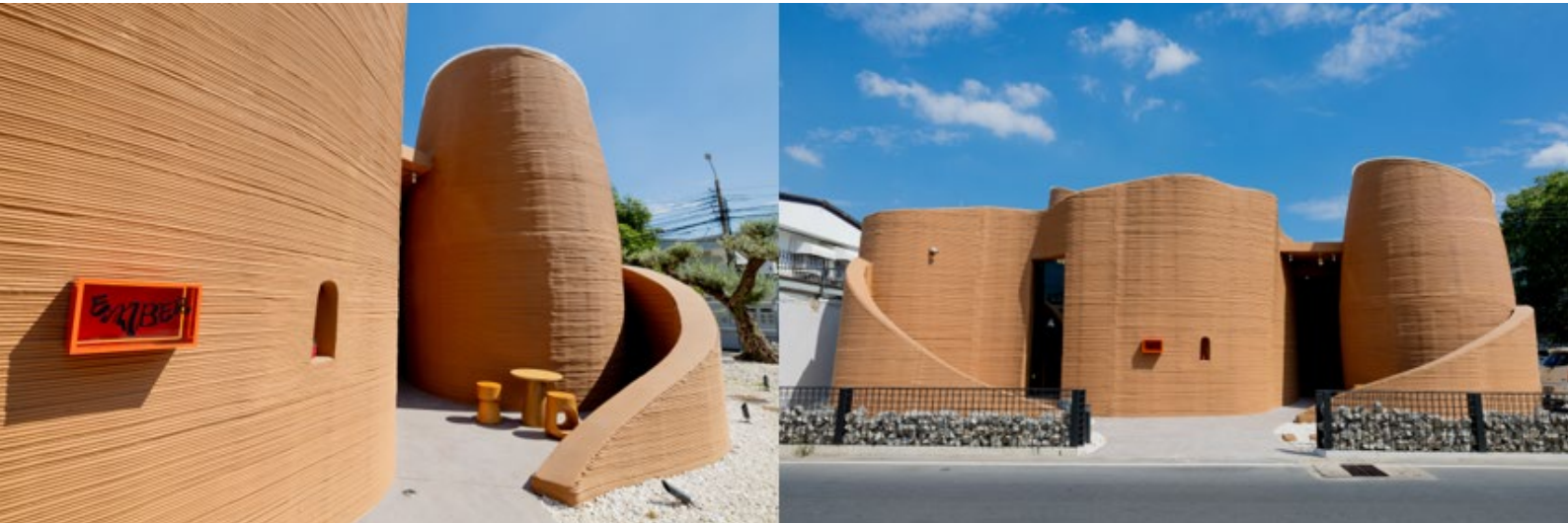
Ember Cafe, located at Rama 9 Soi 43, stands out with its design featuring freeform curves and beautiful aesthetics, made possible by SCG 3D printing technology.
