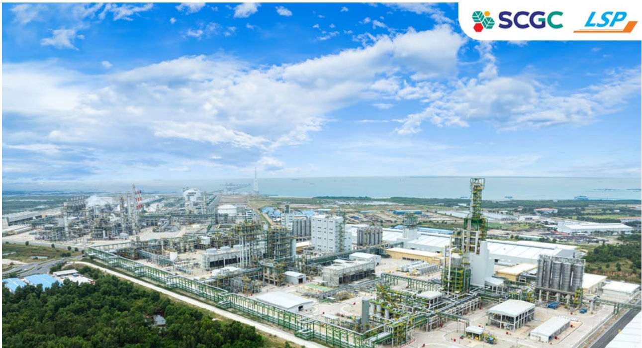
Long Son Petrochemicals (LSP) Project, Vietnam.
